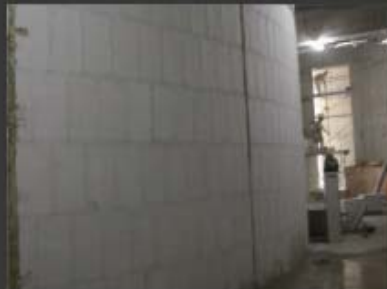
Singapore History Museum plastec light weight blocks can be tilted to achieve a curve wall and still maintaining its strength and rigidity.
