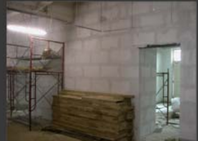
Majestic Hotel with plastec light weight block wall system.(with insulation)
