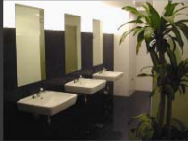
Marina Square toilet Wall tiles is easily installed with normal tile adhesive. Wall hung basin and urinal fix on plastec light weight block.
