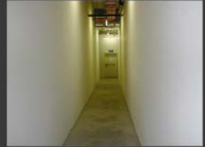
Marina Square fire escape corridor. Its smooth, straight and evenness proved it to be an excellent product for a 4 hours fire rated block.
