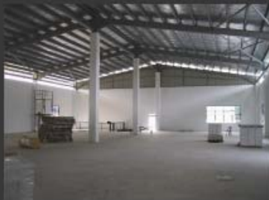
2 Storey Factory at Sungei Kadut. External and internal wall system.
